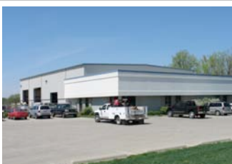
METAL BUILDING WITH EFIS FACADE
